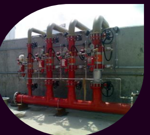
• Sprinkler Control Valve
